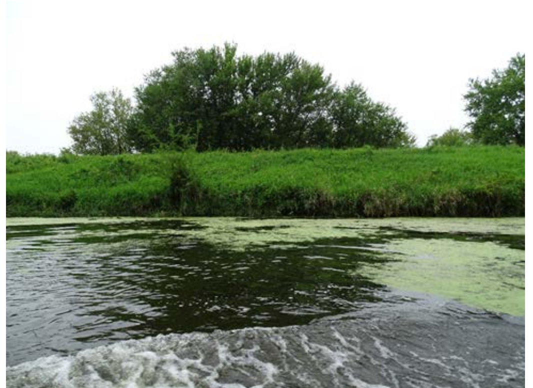
Toe erosion on Green Island levee
