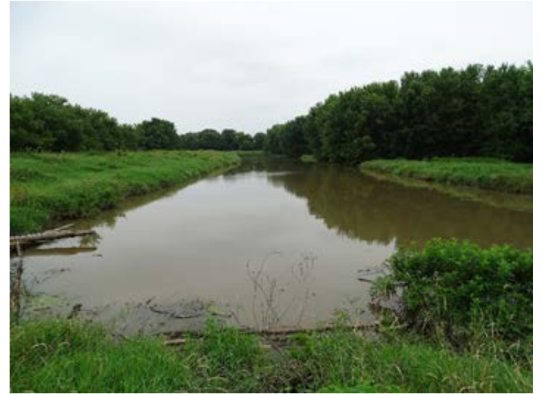
Inlet Channel upstream of WCS
